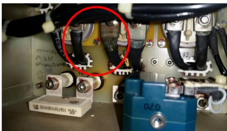
Sign of overheat on relay of the SPC
